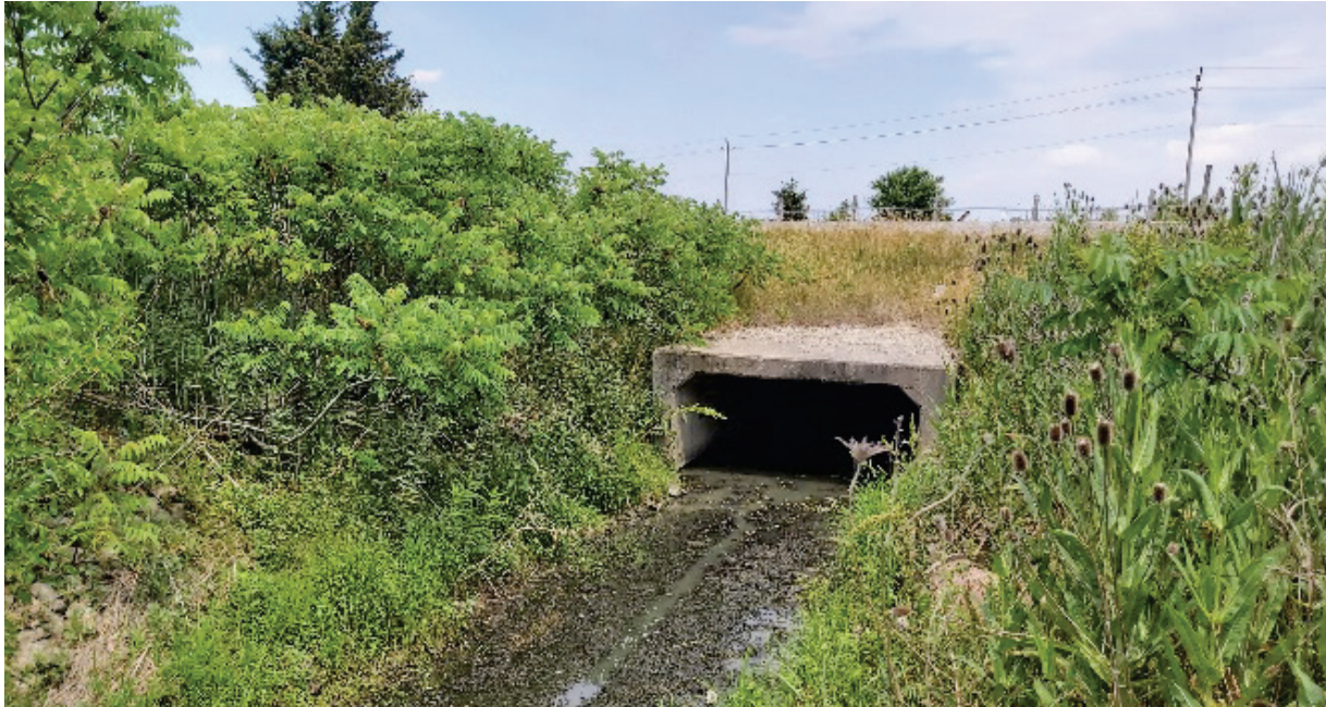
Figure 2-9 Highway 3 Structural Culvert
